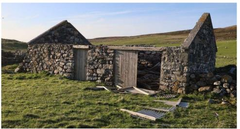
South Elevation: Open joints in stonework, partial wall collapse in south west corner, timber lintels in poor condition, east gable appears to be developing a lean outwards. Photo Sept 24.
