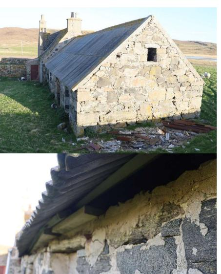
West gable – Open stone joints, settlement and splaying of roof. Loose and broken asbestos cement sheeting.
