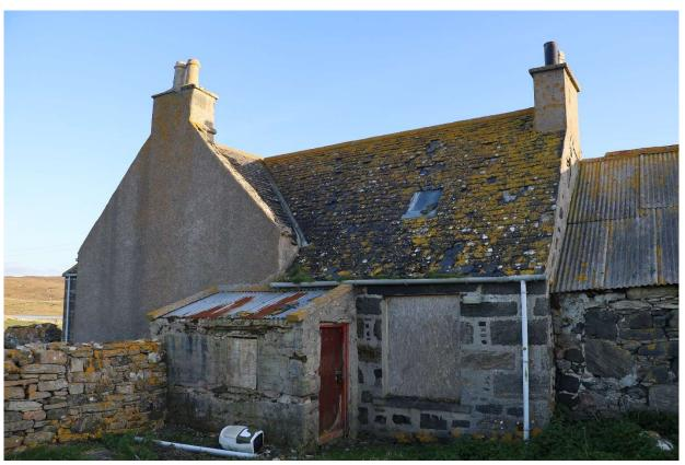
View of NW Corner. Many missing slates with exposed sarking, no under slate membrane, loose slates blocking the valley gutter, skews eroded, west gable poor and open pointing, more recent porch addition in very poor condition.
