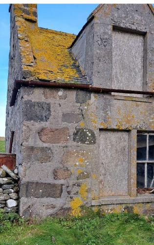
There is cracking in the northwest and southeast walls of the original 1820's house close to the south west gable. While the cracking is not significant it does indicate some movement in the structure.
