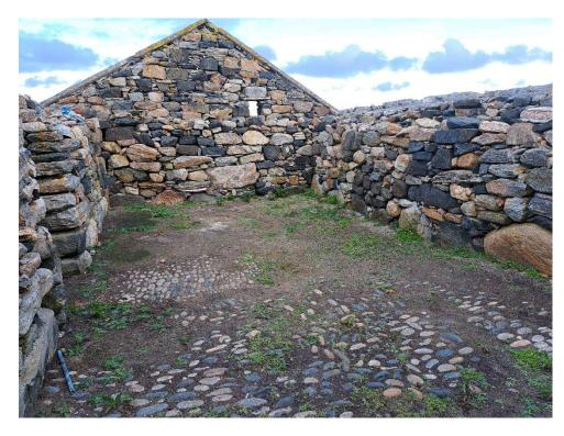
Internal of Byre looking west showing open joints in stonework and cobble floor. Photo Sept 24.
