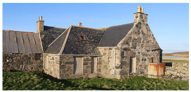
View of SW Corner. Many missing slates with exposed sarking, no under slate membrane, loose slates blocking the valley gutter, skews very eroded, vegetation in valley gutters, pointing in poor condition on south gable elevation and west facing wall of original house, cracking in gable on line of flues. The chimney cope, on the north east side of the chimney on the south west gable has partly broken or eroded away. The stone below is also badly eroded.
