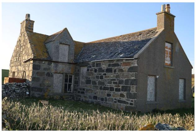
View of SE Corner. (The original house has the gable window.) Many missing slates with exposed sarking, no under slate membrane, loose slates blocking the valley gutter, skews very eroded, loose pointing at skews, gutters partly collapsed, cracking at lintel in 1890-1904 extension.
