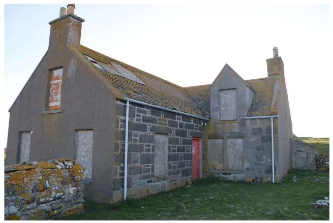
View of NE Corner. (The original house has the gable window.) Extensive area of slate missing from the east 1890-1904 extension, slates missing from the original house, no under slate membrane, loose slates blocking the valley gutter, skews eroded, east gable rendered.
