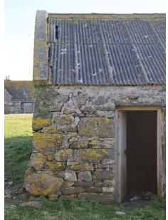
North elevation east end – Extensive cracking in wall and roof sheeting caused by movement in the east gable.
