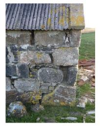
North East Corner – Open stone joints, missing stones, rotation of large stone on second course on gable, possible location of corner base stone, no evidence of any foundation. Loose and broken asbestos cement sheeting.
