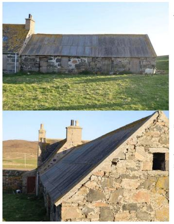
North Elevation – Dipping in ridge line showing the settling and splaying in the roof.
