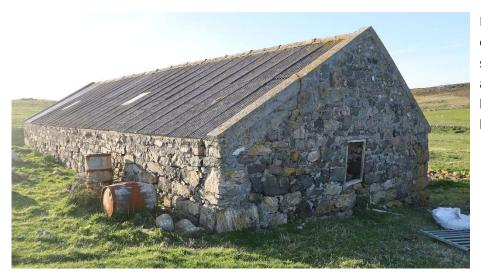
East gable and south elevation. Sand build up to south a west. Floor level is at the north side of the building. Cracking and bulging of east gable.
