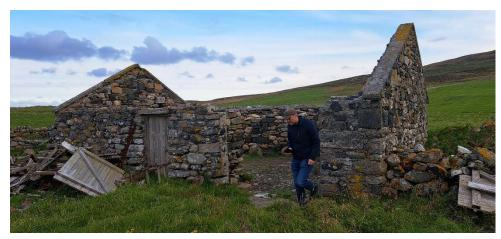
Since the first inspection in May 2019 the complete roof of this building has collapsed along with the larger door and lintel above. The collapsed roof, which contained asbestos cement sheeting, has been removed from
