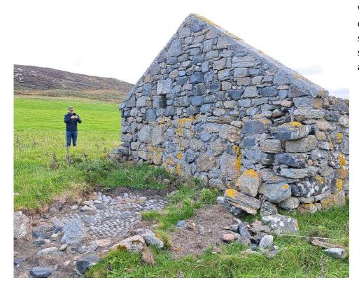
West elevation showing open joints in stonework, loose stonework in SW corner and area of cobble floor.
