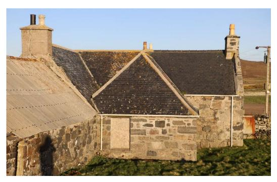
North west elevation showing missing slates, blocked valley gutters, sever cracking in chimney and settlement of the adjoining byre roof.
