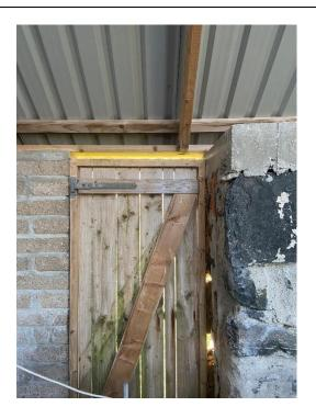
Photograph 16 – Building C: truss end onto wall head with no supporting lintol under
