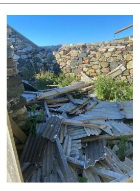
Photograph 8 – Building B: Roof remnant and tiles within footprint
