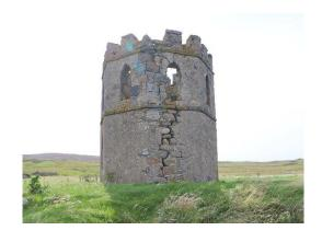
Photograph 36 – Significant cracking, lean and stone displacement to north elevation
