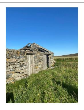
Photograph 7 – Building B: Note wall condition and roof collapse
