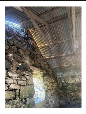
Photograph 19 – Building D: Internal view to gable (note relatively new timber and relatively open jointed masonry)
