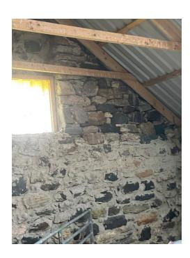
Photograph 18 – Building D: possible roof separation at gable
