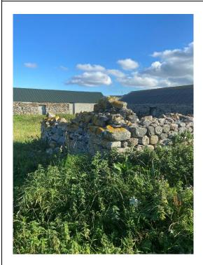
Photograph 3 – Building A: corner with generally loose stone
