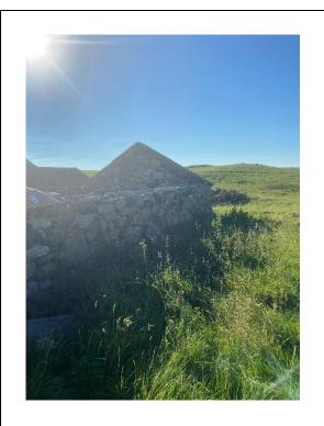
Photograph 9 – Building B: Unrestrained gable and unprotected wall head
