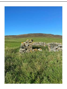
Photograph 5 – Building B: wall remnants, note high and loose stones
