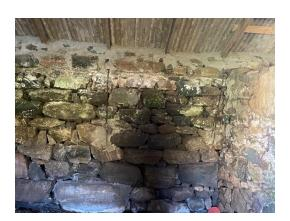
Photograph 20 – Building D: Bootlace tie straps pocketed into wall
