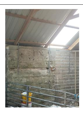
Photograph 15 – Building C: trusses tied down to concrete infill wall
