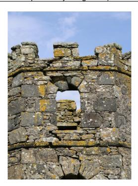
Photograph 39 – Typical key stone displacement
