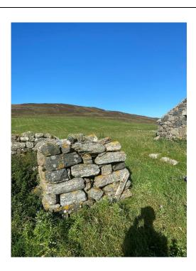
Photograph 6 – Building B: corner with loose stones
