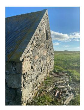
Photograph 25 – Note dip in byre roof and large crack in chimney flue
