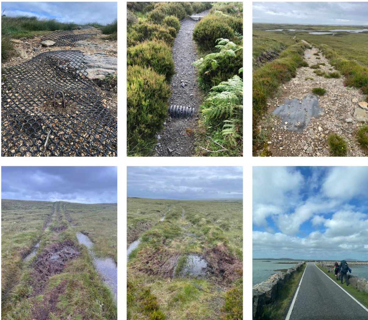
Figure 10: Images of the Hebridean Way path between Carinish & Langass Woodland on North Uist as an illustration of the current condition and dangers _ c Fraser Architecture LLP 2022.
