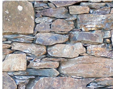
Reinstated Dry Stone Wall
