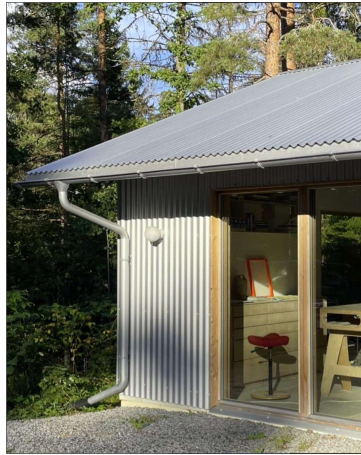
Metal sheet roof
