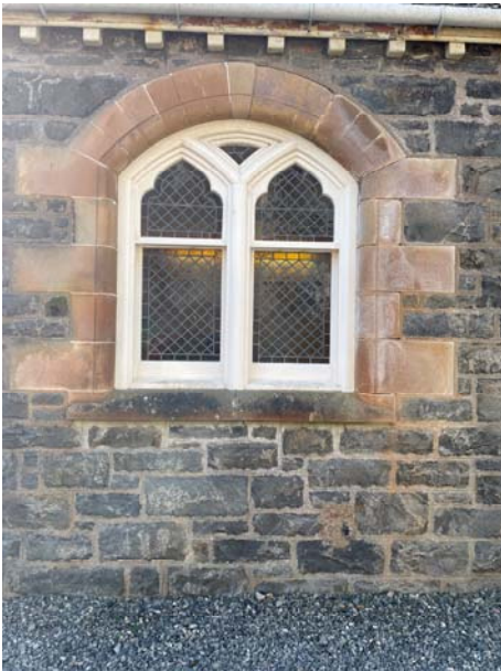
Photo 1. Existing window in east elevation to be Removed and opening extended to ground level To allow a new external entrance door to be Installed. The design of the upper part of the Window is to be retained for the screen above the Proposed new door.
