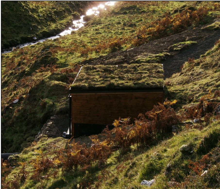
Figure 6: Example Turbine House (Isle of Skye).
