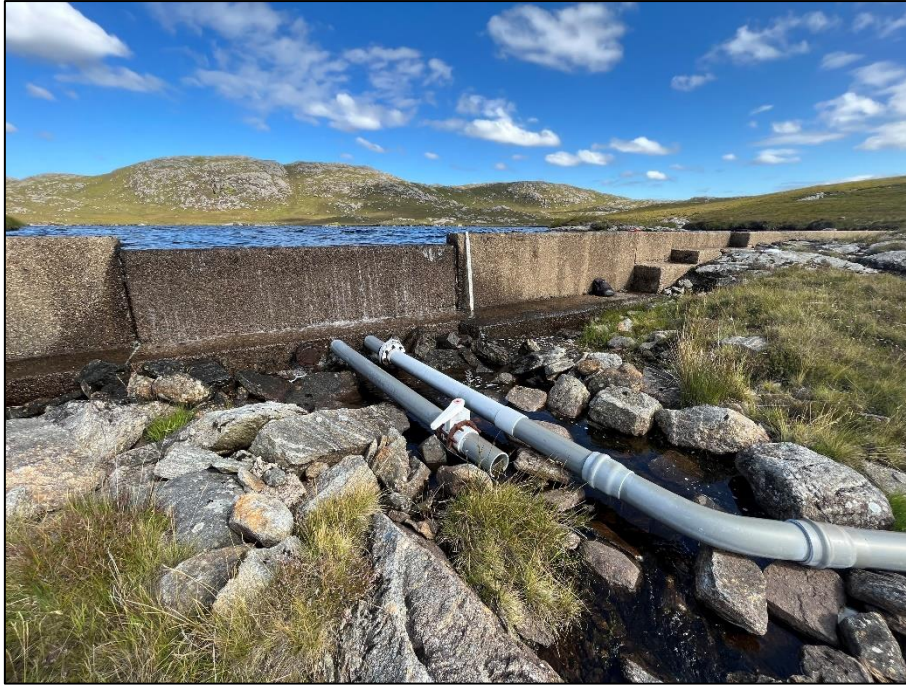
Figure 2: Existing abstraction location.
