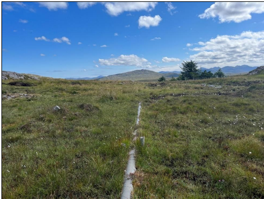
Figure 3: Typical Topography in upper section of penstock route alongside the existing penstock which is visible.
