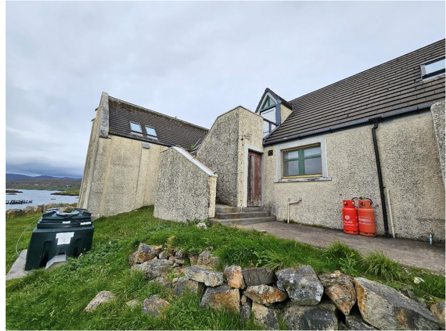
VIEW 6: showing the rear entrance of the Community Centre to the west of the building.
