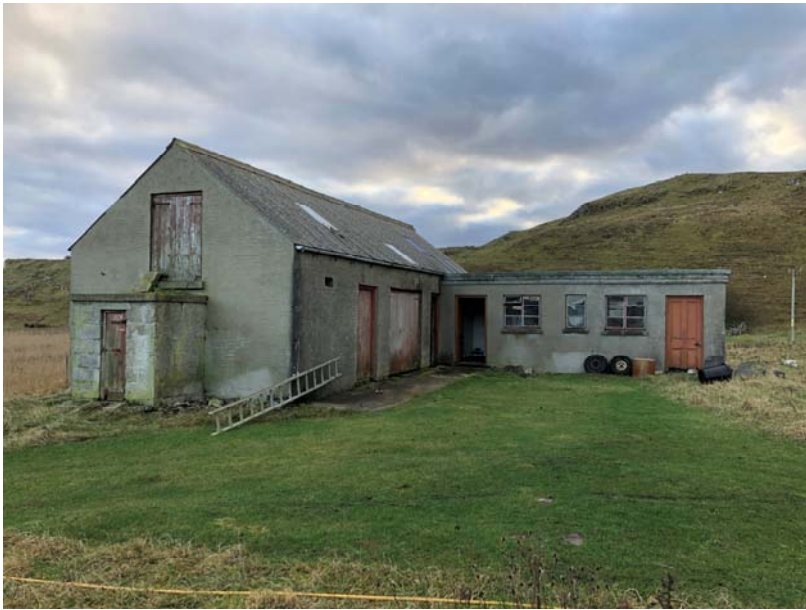
Image 2. The existing barn, to be demolished.
