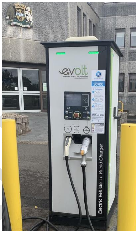
Fig. 3 - 43kW/50kW Charging Point at Western Isles Council
