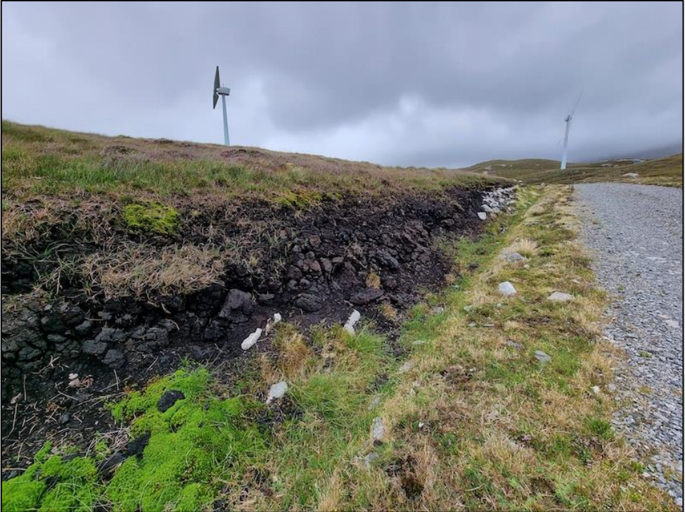
Figure 3: Exposed bare peat along a ditch edge.
