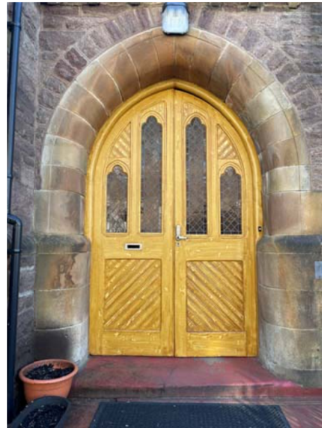
Photo 2. Existing Francis Street door (North Elevation) Deign of new east elevation door to replicate the design of the existing door.
