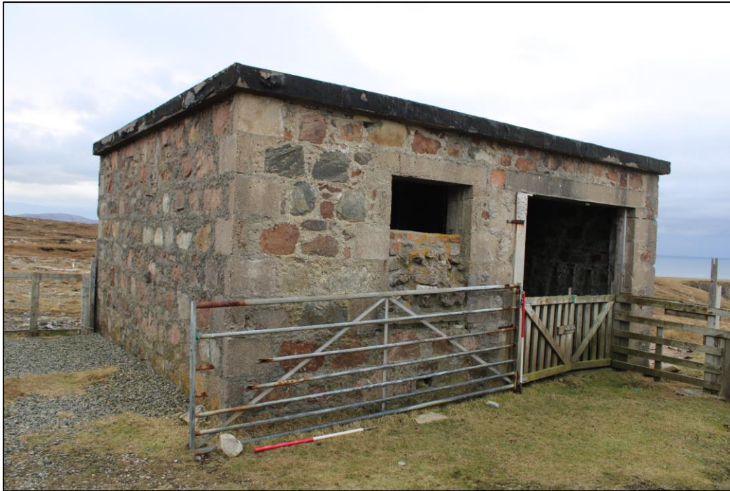
Figure 14: Feature 39, generator block
