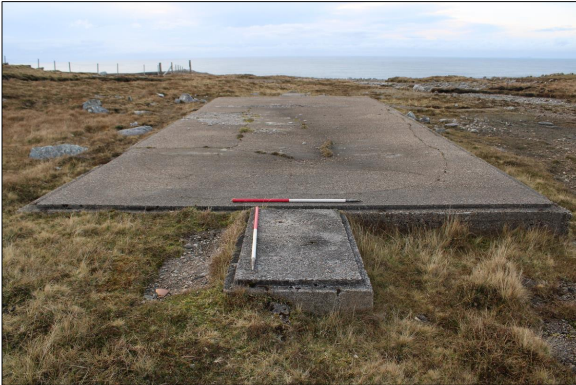
Figure 7: F2 Nissan hut with entrance platform and construction recess.
