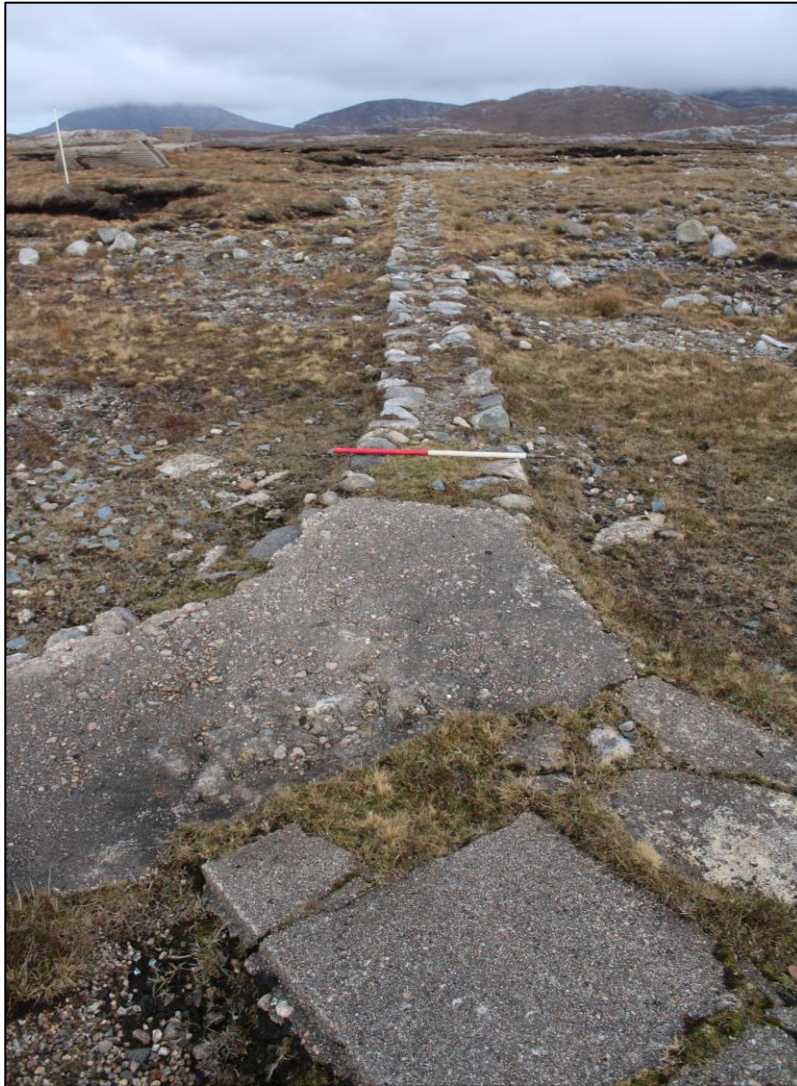
Figure 8: Feature 9 concrete and stone path leading to bunker
