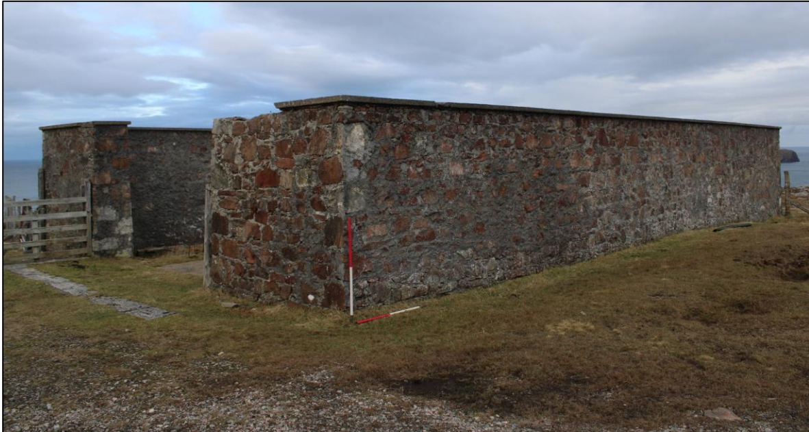
Figure 13: Feature 38, blast walls and transmitter building
