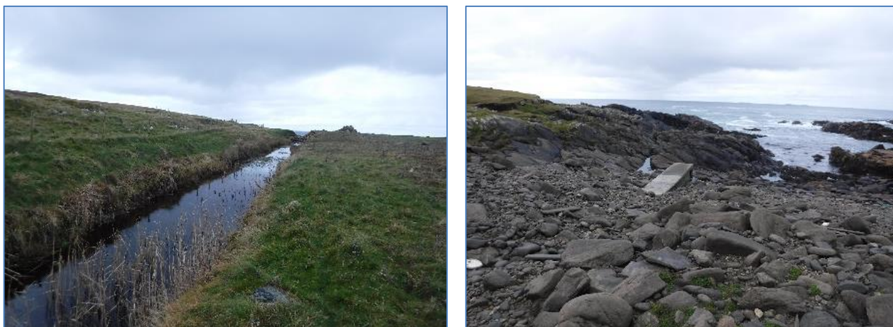
Image 17-2 Discharge outlet of Loch Scolpaig and associated drainage channel.
