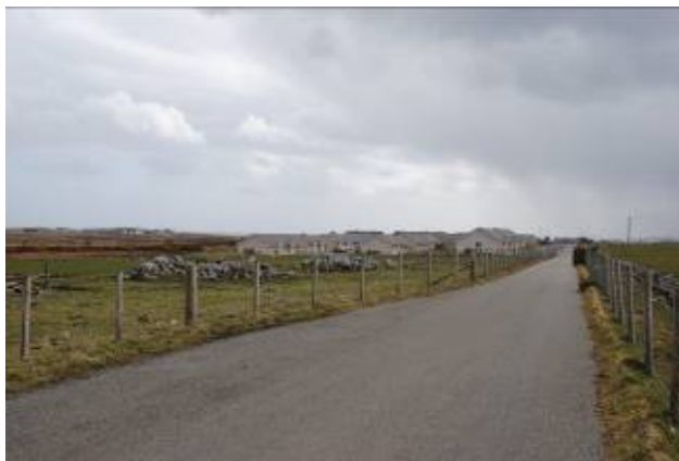
Fig 12 Main spine road on site
