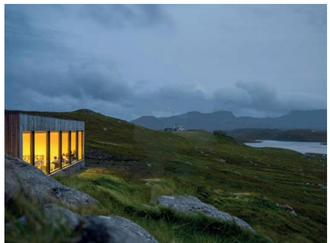
Uig Sands restaurant by Dualchas on the Isle of Lewis – simple form with weathered timber.
