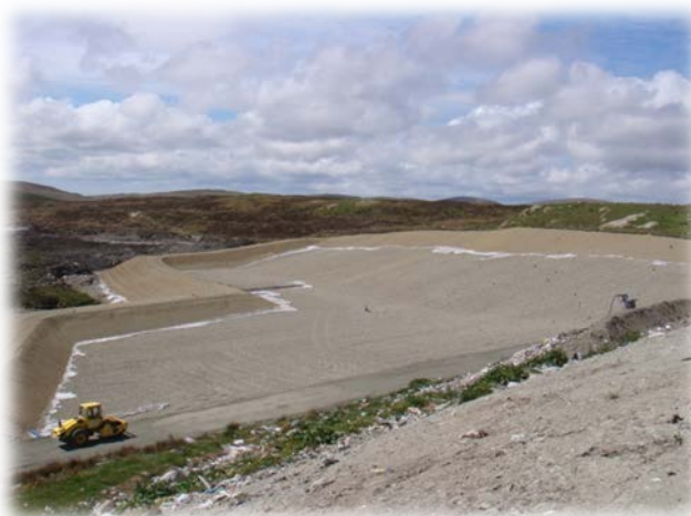
Figure 2 New Landfill Extension at Bennadrove - June 2012
