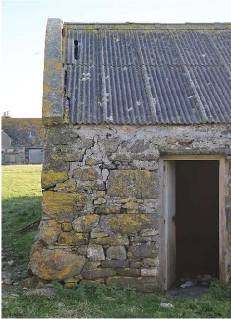
North elevation east end – Extensive cracking in wall and roof sheeting caused by movement in the east gable.
