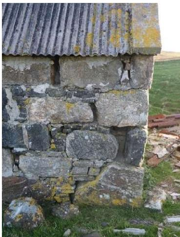
North East Corner – Open stone joints, missing stones, rotation of large stone on second course on gable, possible location of corner base stone, no evidence of any foundation. Loose and broken asbestos cement sheeting.
