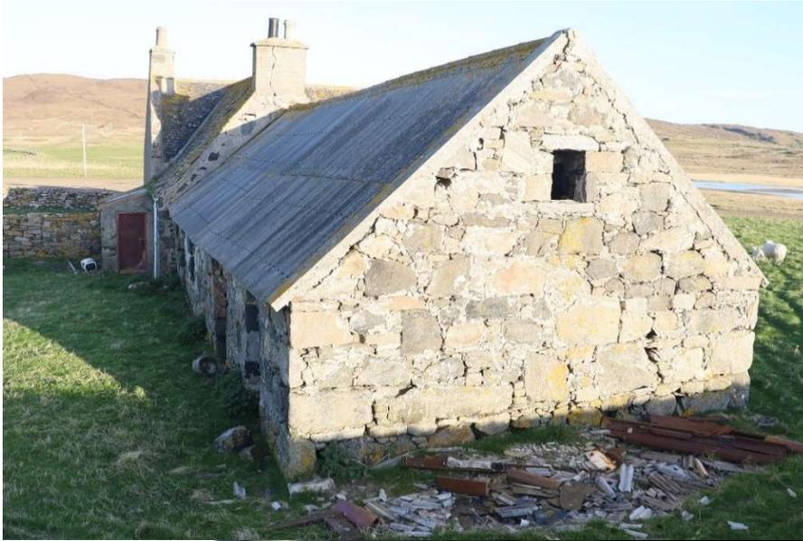
West gable – Open stone joints, settlement and splaying of roof. Loose and broken asbestos cement sheeting.
