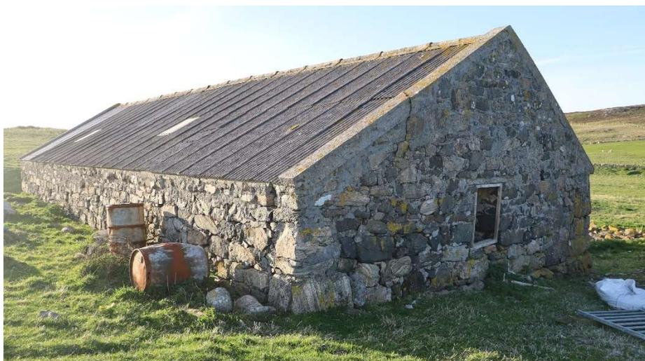
East gable and south elevation. Sand build up to south a west. Floor level is at the north side of the building. Cracking and bulging of east gable.
