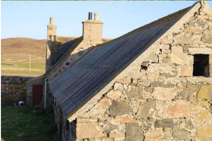
North roof and west gable – Settlement and splaying in roof clearly evident. Note gap between the pointing on the house gable and roof sheeting. Skew badly cracked upper stone walls dislodged. Open pointing in gable stonework.
