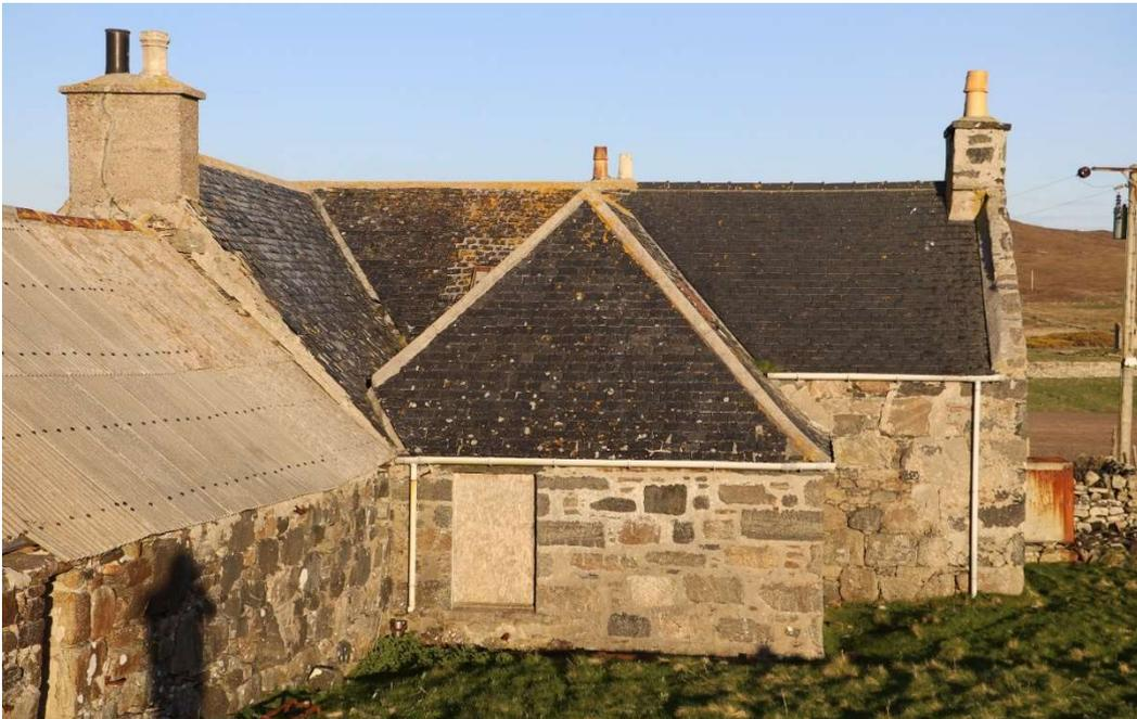
North west elevation showing missing slates, blocked valley gutters, sever cracking in chimney and settlement of the adjoining byre roof.
