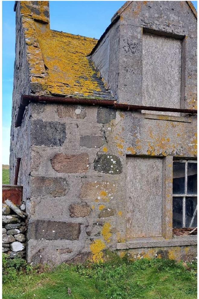
There is cracking in the northwest and southeast walls of the original 1820's house close to the south west gable. While the cracking is not significant it does indicate some movement in the structure.
