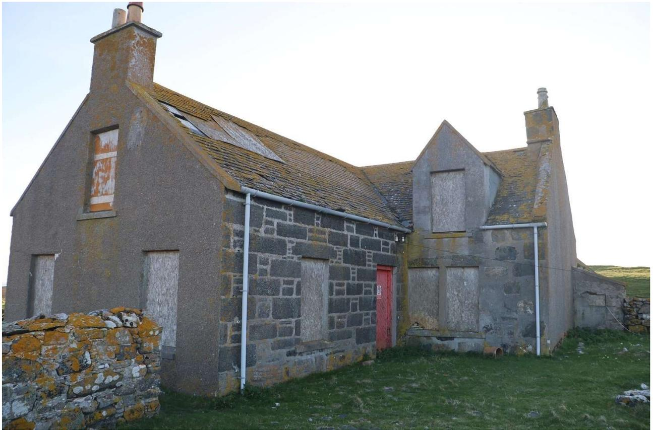
View of NE Corner. (The original house has the gable window.) Extensive area of slate missing from the east 1890-1904 extension, slates missing from the original house, no under slate membrane, loose slates blocking the valley gutter, skewers eroded, east gable rendered.
