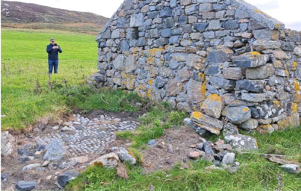
West elevation showing open joints in stonework, loose stonework in SW corner and area of cobble floor.
