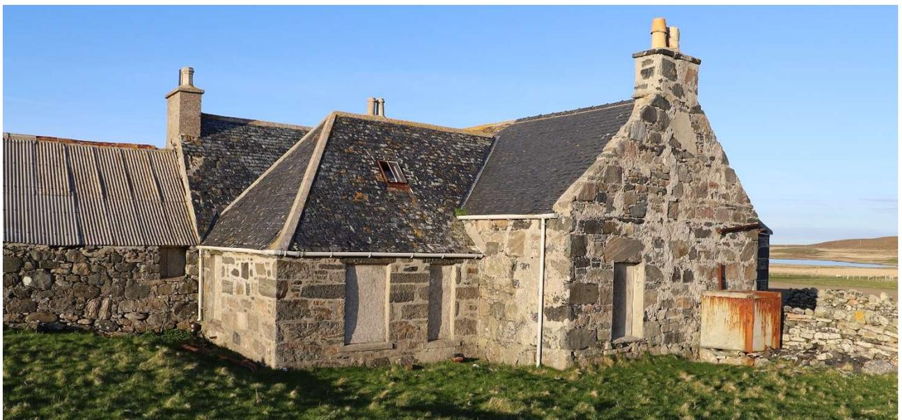
View of SW Corner. Many missing slates with exposed sarking, no under slate membrane, loose slates blocking the valley gutter, skewers very eroded, vegetation in valley gutters, pointing in poor condition on south gable elevation and west facing wall of original house, cracking in gable on line of flues. The chimney cope, on the north east side of the chimney on the south west gable has partly broken or eroded away. The stone below is also badly eroded.
