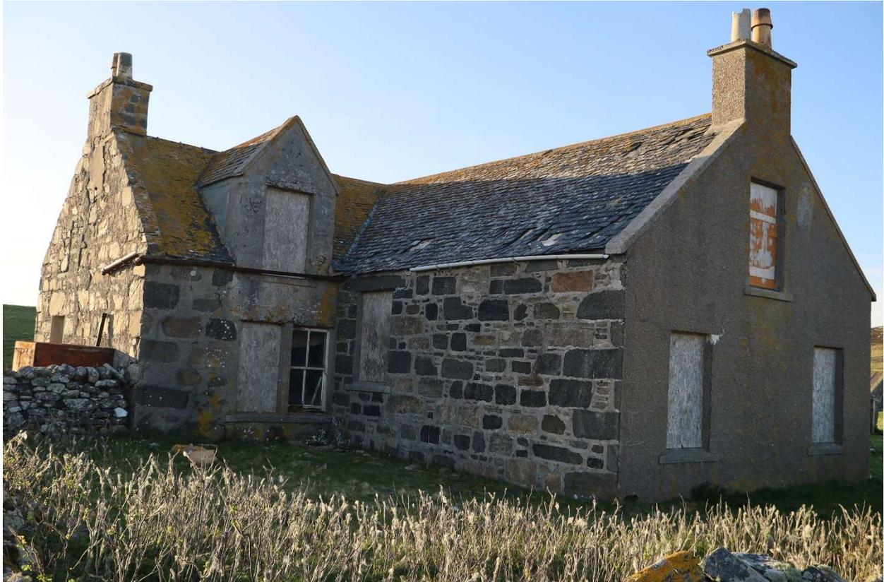
View of SE Corner. (The original house has the gable window.) Many missing slates with exposed sarking, no under slate membrane, loose slates blocking the valley gutter, skewers very eroded, loose pointing at skewers, gutters partly collapsed, cracking at lintel in 1890-1904 extension.
