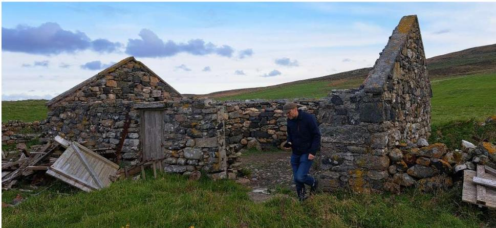
Since the first inspection in May 2019 the complete roof of this building has collapsed along with the larger door and lintel above. The collapsed roof, which contained asbestos cement sheeting, has been removed from
