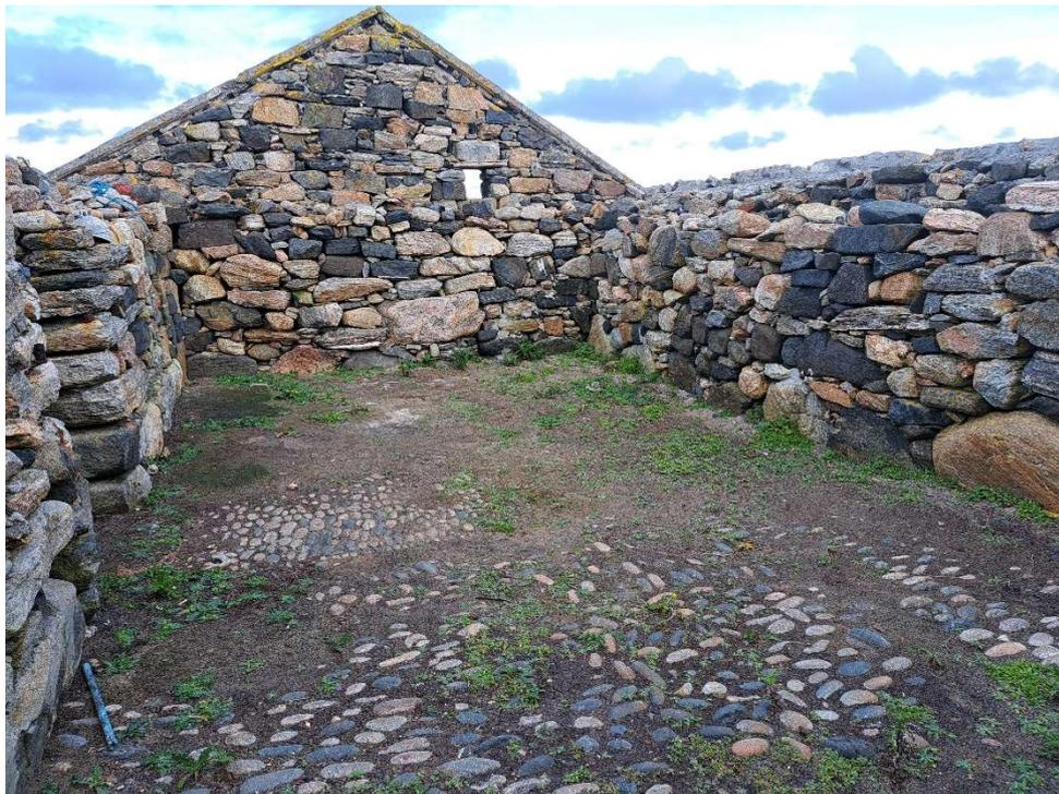
Internal of Byre looking west showing open joints in stonework and cobble floor. Photo Sept 24.
