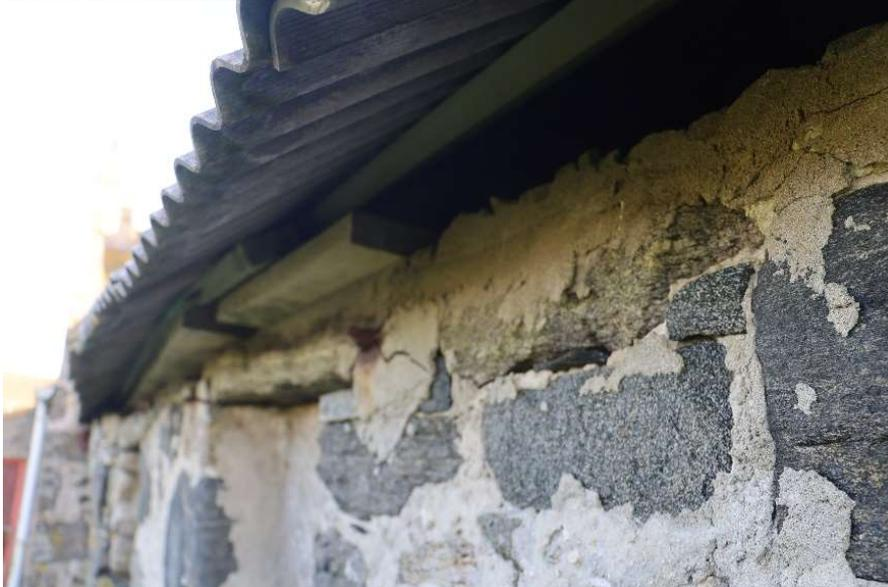
Eaves, North Elevation – Settlement of roof pushing support structure out beyond the wall head.
