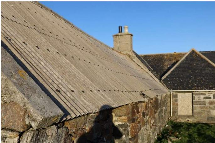
South roof and wall. - Settlement in roof clearly evident. Note gap between the pointing on the house gable and roof sheeting. Bulging in stone walls.
