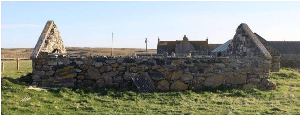
North Elevation: Open joints in stonework, roof debris including broken asbestos cement sheeting and timber. Photo May 24.
