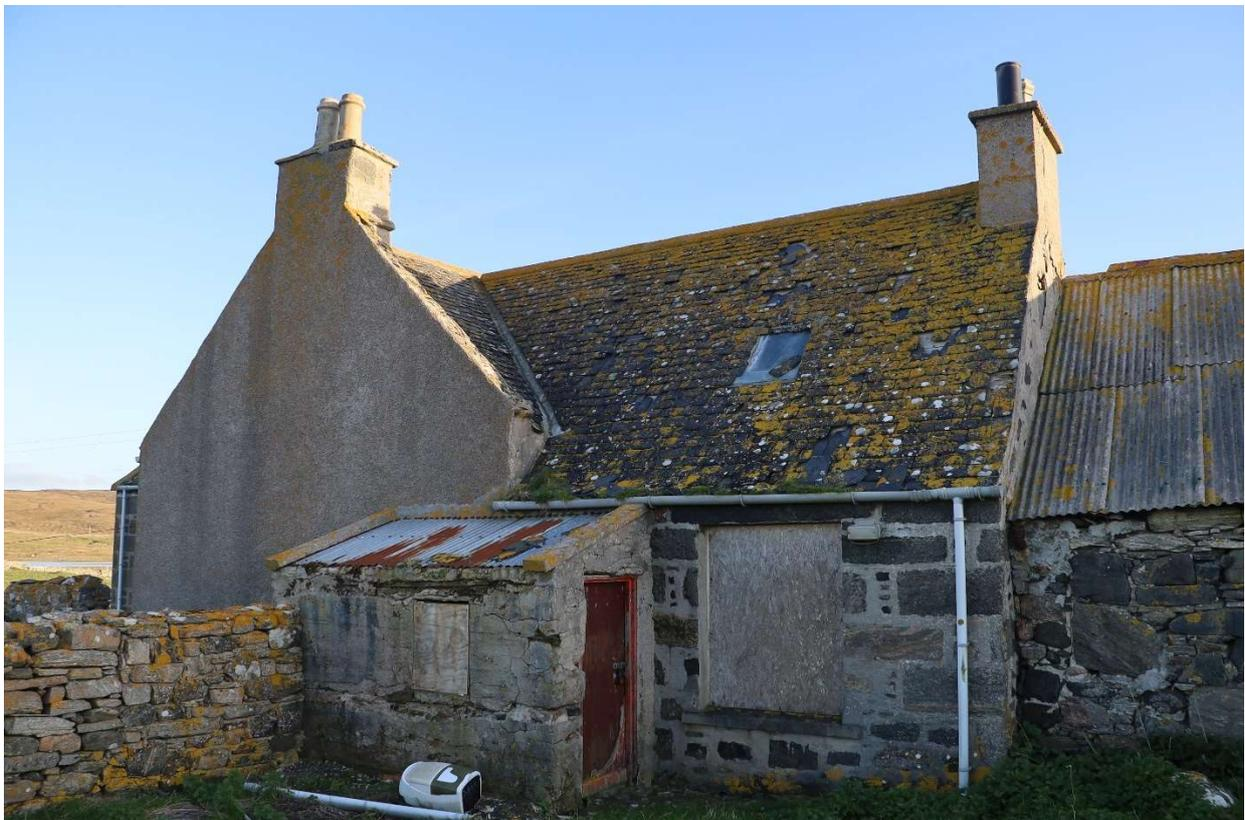
View of NW Corner. Many missing slates with exposed sarking, no under slate membrane, loose slates blocking the valley gutter, skewers eroded, west gable poor and open pointing, more recent porch addition in very poor condition.
