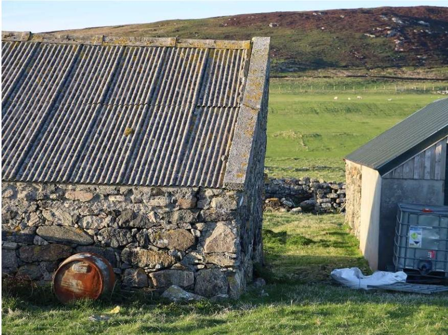
South elevation showing cracking, bulging and distortion in east gable. Cracked to skew.
