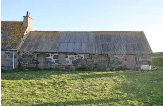
North Elevation – Dipping in ridge line showing the settling and splaying in the roof.
