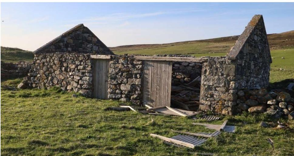
South Elevation: Open joints in stonework, partial wall collapse in south west corner, timber lintels in poor condition, east gable appears to be developing a lean outwards. Photo Sept 24.
