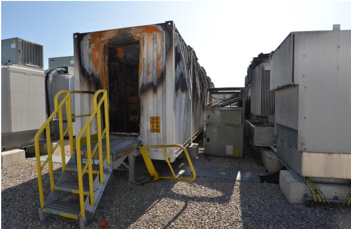
Image above: Exterior of unit with pressure damage to side.
