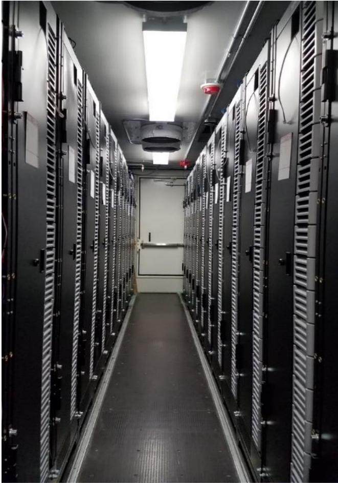
Note configuration of lithium ion banks, narrow access corridor and cooling vents fitted to ceiling.
