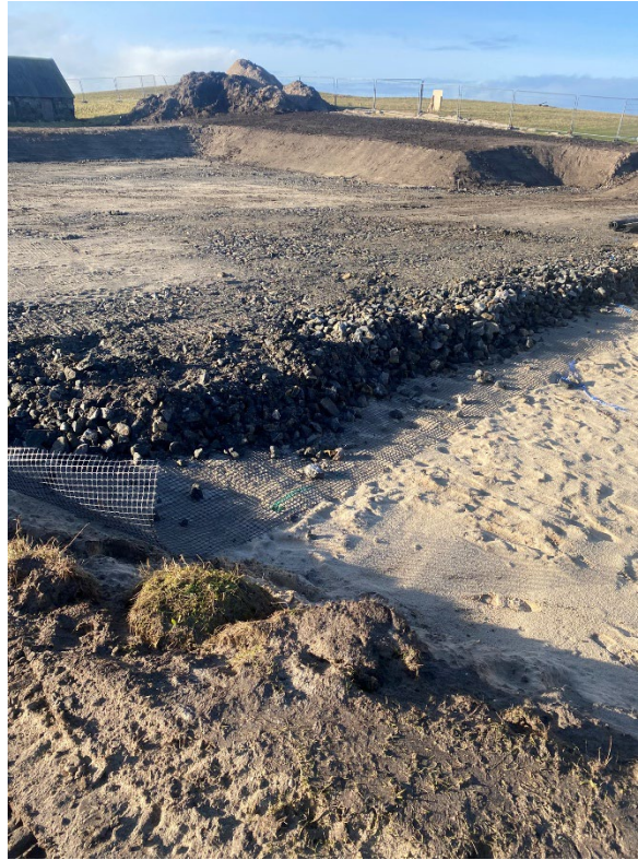
Photo 6 Silt mitigation measures
