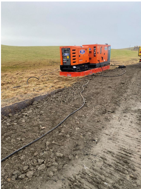
Photo 5 Pump generator containment systems
