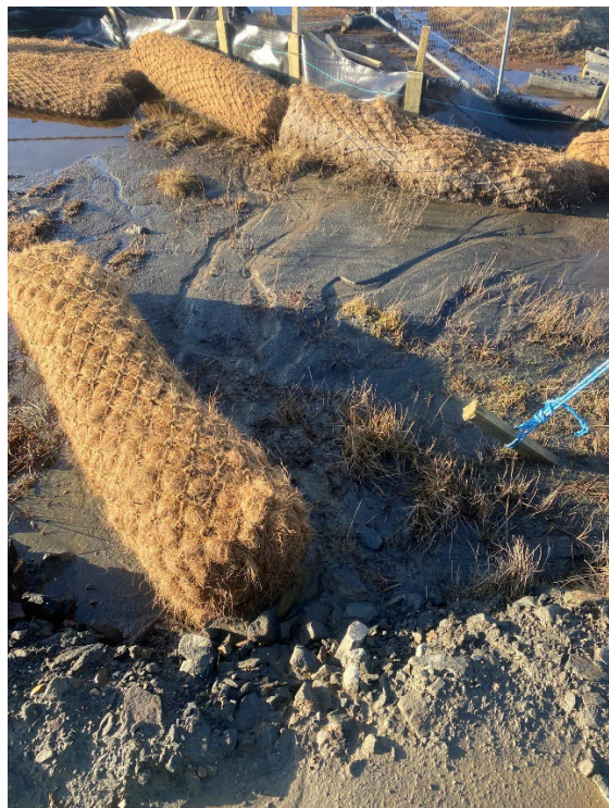
Photo 6 Silt mitigation measures
