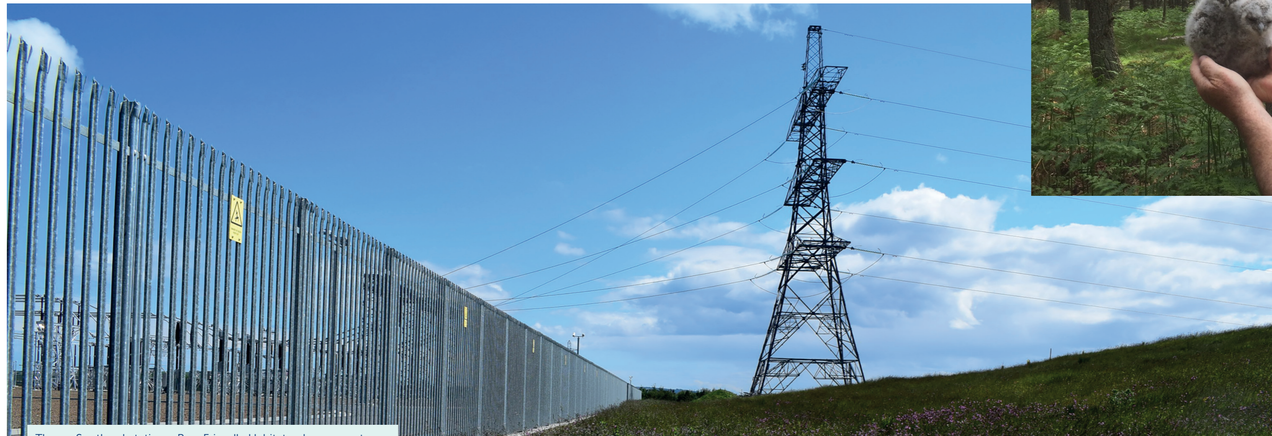
Thurso South substation - Bee-Friendly Habitat enhancement area
