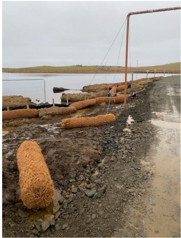
Photo 8 Extensive silt mitigation measures
