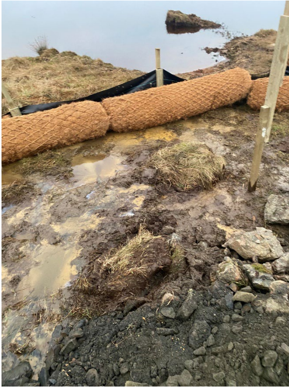
Photo 7 Silt mitigation measures
