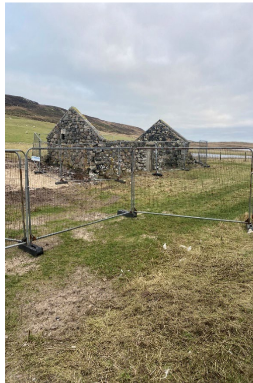
Photo 10 Fencing around heritage sites
