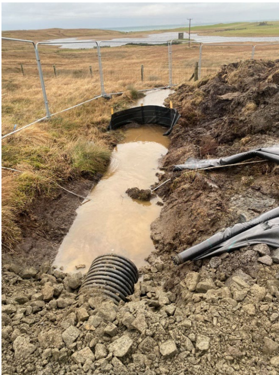
Photo 1 New culvert feeding under the A865
