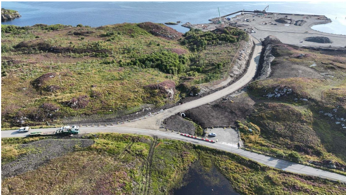
Figure 2.1: DWP and Access Road Under Construction (September 2023)
