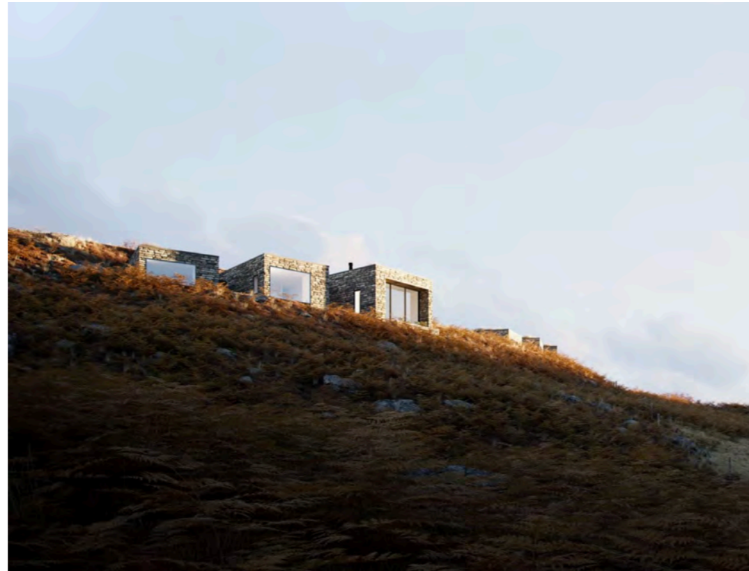
2 houses at Portnalong, Skye, Scotland, Dualchas Architects
