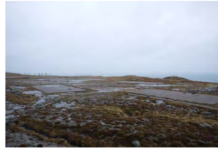
B - Concrete Pads
