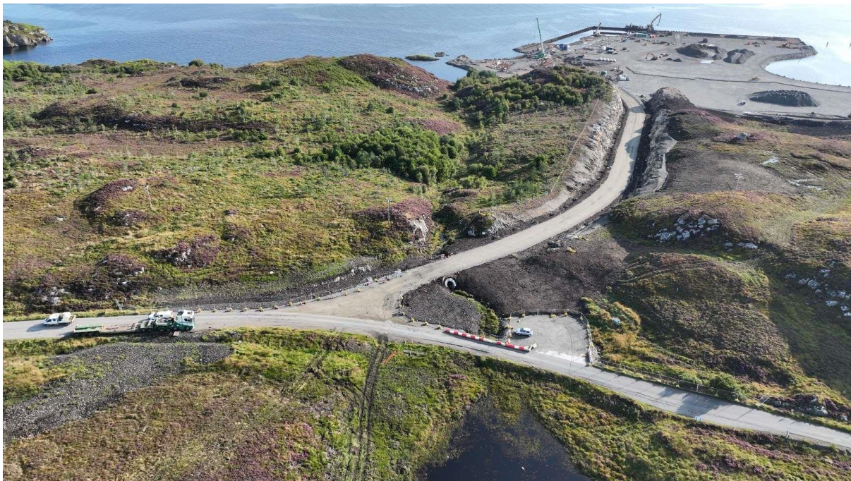
Figure 2.1: DWP and Access Road Under Construction (September 2023)
