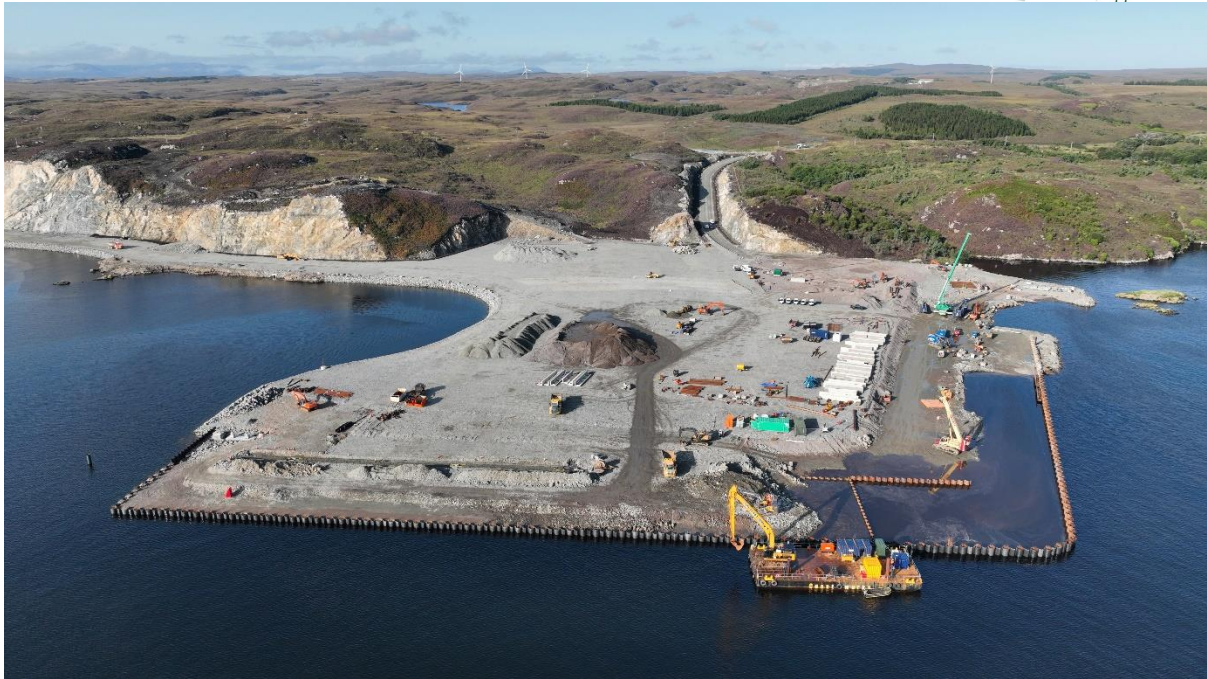
Figure 2.2: DWP Construction Progress (September 2023)
