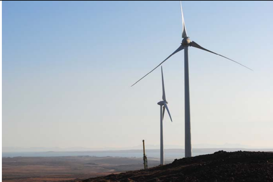
Pentland Wind Farm, Isle of Lewis
